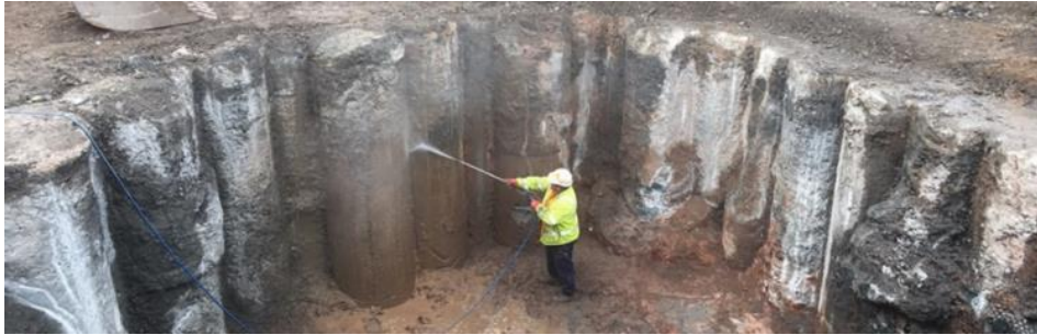
Figure 14. Exposed piles during construction.
